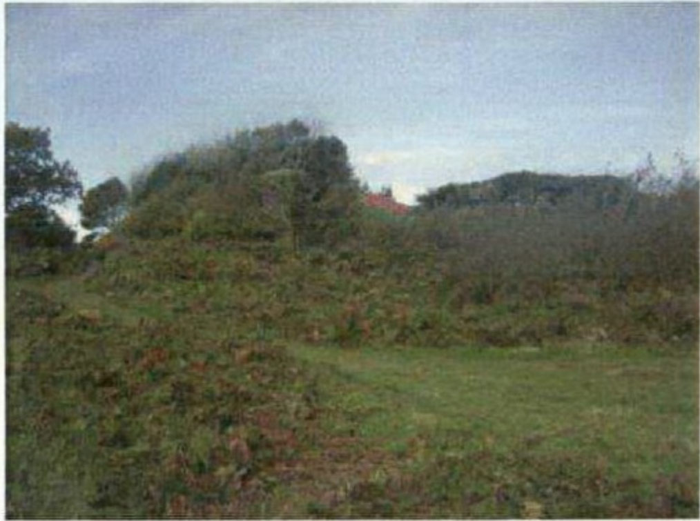
Plate 5: Existing building viewed from south
